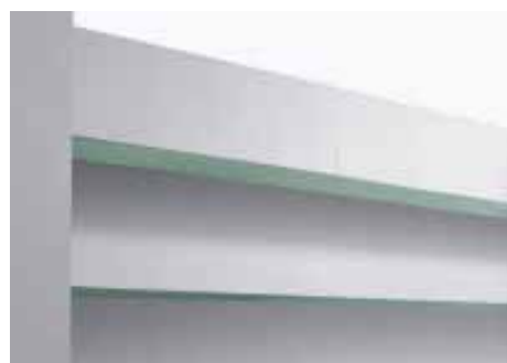
Ablageboard, Glas satiniert 6 mm, Weißglas ESG an Paneelwand gesteckt/ Storage shelf, 6mm satinised glass, clear ESG safety glass on panel wall, rests in groove
